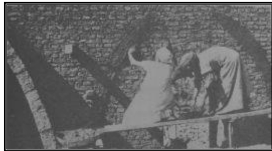
F 3. Second step, forming the curve on the wall using mortar. Place of construction: Egypt (Source: Besenval 2000, Fahi, 2003)
