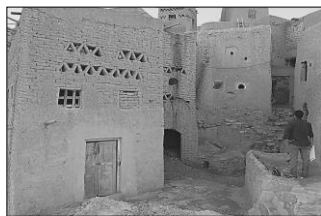
F18. An example of single block houses. Source: Authors.
