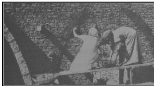
F 3. Second step, forming the curve on the wall using mortar. Place of construction: Egypt (Source: Besenval 2000, Fahi, 2003)
