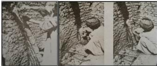
F 4. Third step, forming the curve on the curved line of wall on the back wall. Place of construction: Egypt (Source: Besenal 2000, Fahi, 2003).
