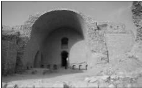
F 8. A barrel vault with buttress, Fire temple of Firouzabad, Fars Province (Source: Negarandegan).
