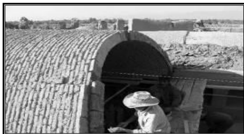
F6. Leveling the vault using ropes. Place of construction: Abarkouh, Yazd Province, vault restoration (Source: Negarandegan).
