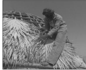
F11. Plover: The leaf of Daz tree (a local tree), which is used to cover the hut.
