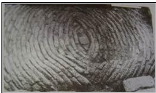
F 7. One of the oldest examples of Lilipoush vaults was constructed in Tell al-Rimah, Iraq. (Source: Besenval 2000: 108).
