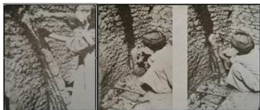
F 4. Third step, forming the curve on the curved line of wall on the back wall. Place of construction: Egypt (Source: Besenval 2000, Fahi, 2003).
