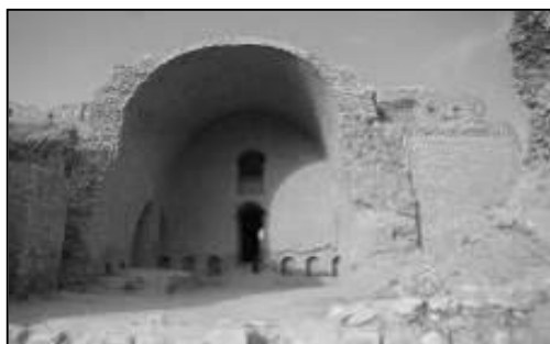
F 8. A barrel vault with buttress, Fire temple of Firouzabad, Fars Province (Source: Negarandegan).
