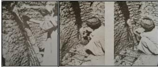
F 4. Third step, forming the curve on the curved line of wall on the back wall. Place of construction: Egypt (Source: Besenal 2000, Fahi, 2003).
